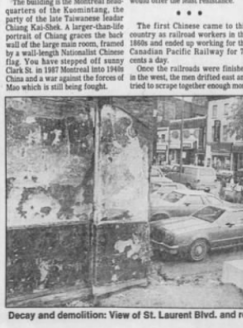
Decay and demolition: View of St. Laurent Blvd. and restaurants from vacant block.
